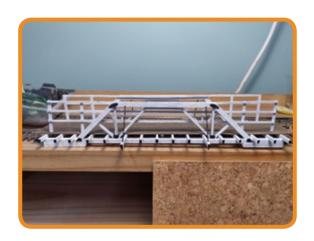
The queen post bridge on the bench. The bridge is scratch built using the original plans from 1868. Timbers in the bridge are true to original dimensions. The largest timbers in the bridge were  $12'' \times 14''$ . The bearers were  $12'' \times 12''$ .
